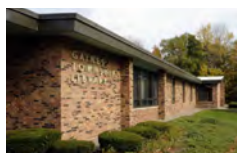
GAINES TOWNSHIP BRANCH 421 68th St. SE Grand Rapids, MI 49548
