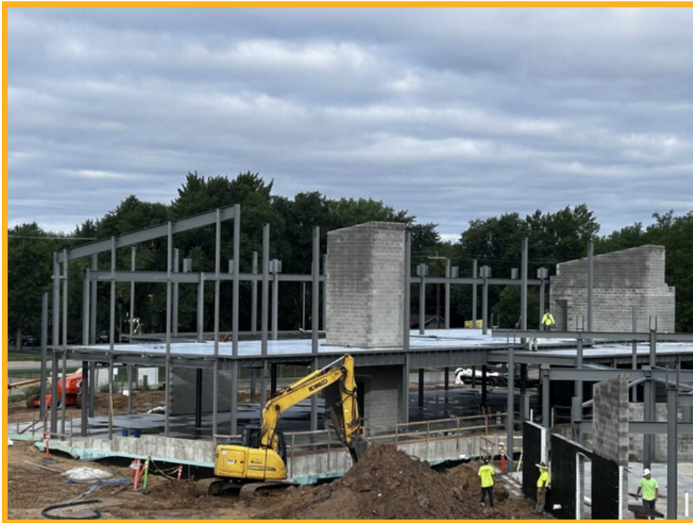
Progress continues on the Walker Expansion
