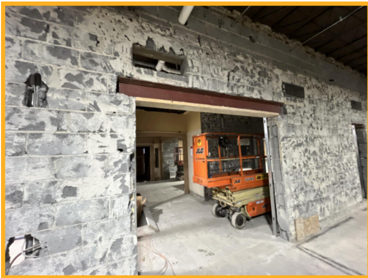
The original building and the addition have now been joined!
