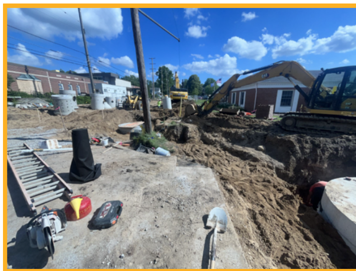
Construction of the plaza is underway
