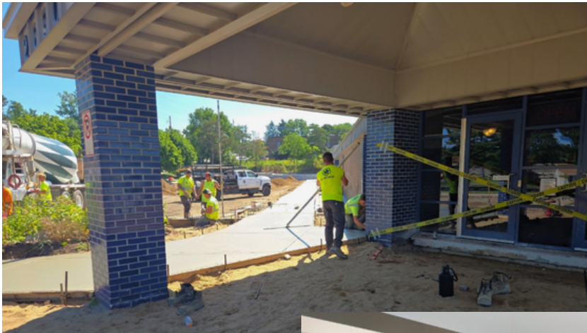
Fresh cement is poured for a main pathway to the Plainfield Branch front entrance.
