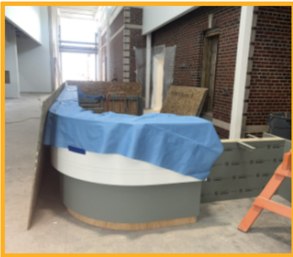
New service desk being installed
